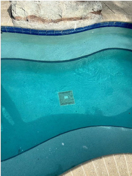
Main Drain – Spa Before
