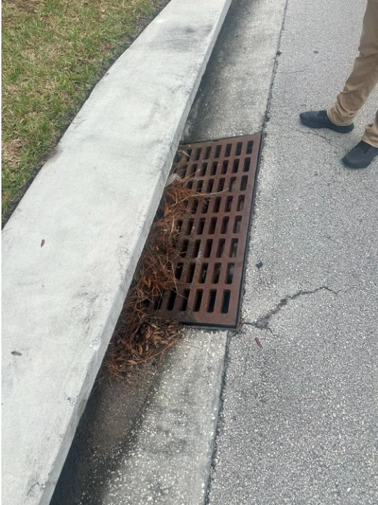
Solterra Blvd Grate - After
